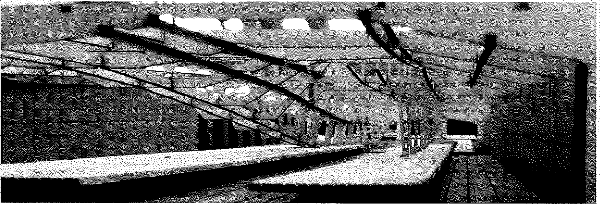
figure_25 Exposed Structure (Platform Level) Çıplak Yapı (Platform Seviyesi)
