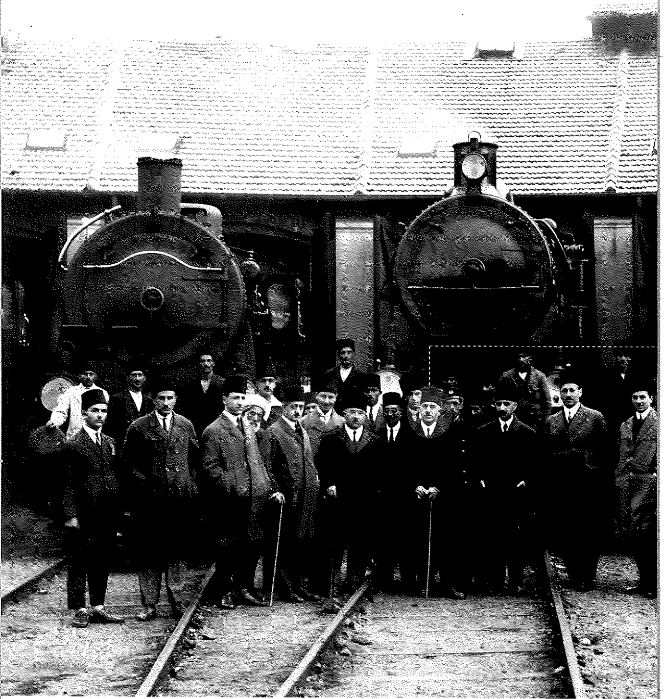
figure_06 Eskişehir Train Maintenance Depot Eskişehir Cer Atölyesi
